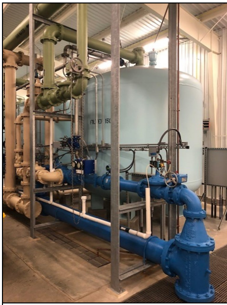
A look at the filter vessels in one of the treatment plants.
