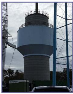
the roof section of the tank. As of this printing, the new million-gallon elevated water tank in West Dennis is structurally complete. With weather hampering further progress on the internal components and final painting, work will resume and be completed this spring. We are pleased to report the project is on-time
