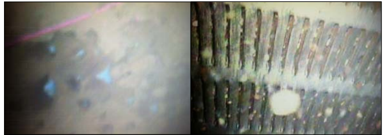
Submerged cameras take before and after pictures for comparison. Routine cleanings improve motor efficiency and increase production.
