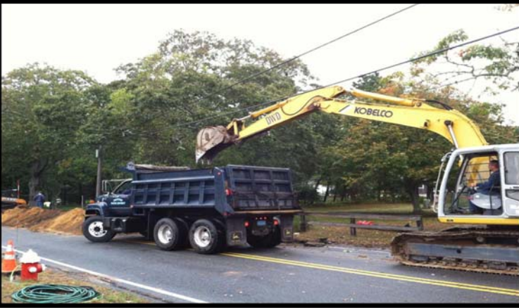
Due to the location of other utilities, it was necessary to place most of the new main within the existing roadway. A temporary patch was put down until the disturbed areas settle, then final road repairs will be made this Spring.
