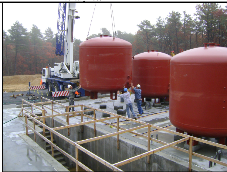
Construction workers help guide the setting of one of six pressure filter vessels hoisted into place by a crane. The six vessels will be capable of removing iron and manganese from 4,000,000 gallons of water per day. The vessels are filled with Greensand Plus filtration media.
