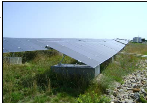
Photovoltaic panels use solar cells to convert energy from the sun into a flow of electrons.
