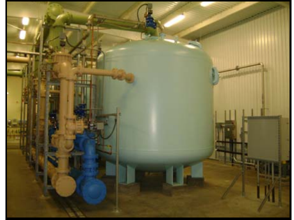
Iron & Manganese Filtration Vessels
