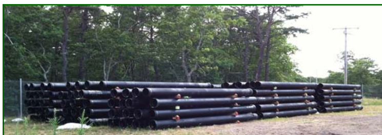
5,000' of 12" water main are stockpiled for installation on Depot Street
