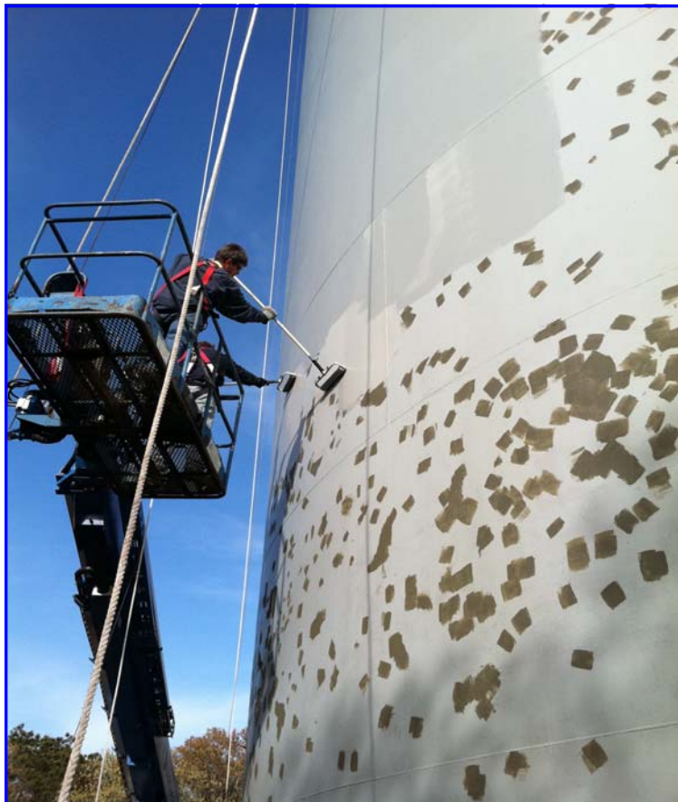
Asst. Superintendent Jim Ritchie and System Maintenance employee Jon Moore apply paint over patched areas known as "stone bruises".
