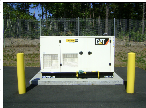
100 kw Standby Generator—Station #21
