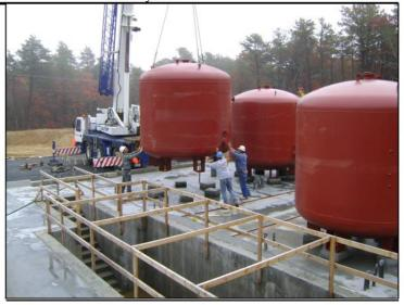
Construction workers help guide the setting of one of six pressure filter vessels hoisted into place by a crane. The six vessels will be capable of removing iron and manganese from 4,000,000 gallons of water per day. The vessels are filled with Greensand Plus filtration media.
